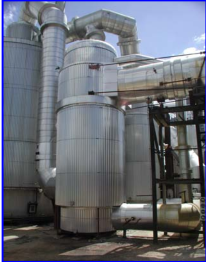
Cold Exchanger Installed
