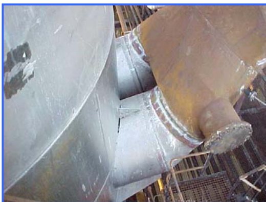
Ducting fit up at Final Tower
