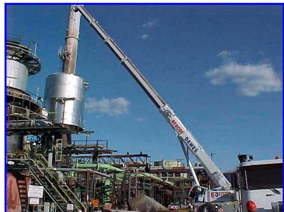
New Final Tower being lifted into position
