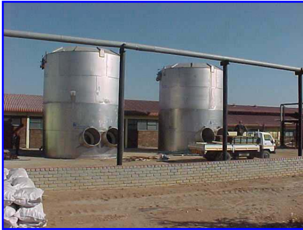
Completed Towers ready for installation
