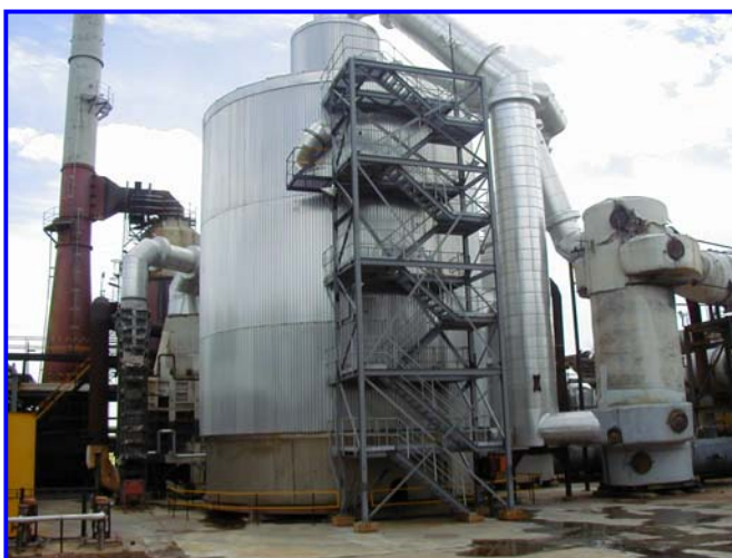
New Converter & ducting installed & operating
