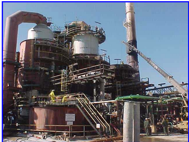
Dismantling Final Tower
