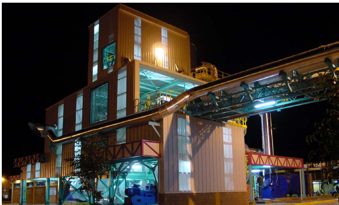
Fig. 5 – WSA plant at a Molybdenum Roasting Plant at Molymex, Mexico
