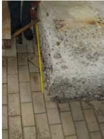
Damaged concrete areas
