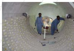
Bricklining under process
