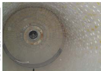
Bricklining job finished
