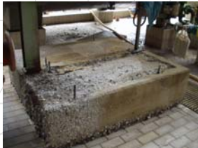
Damaged concrete areas
